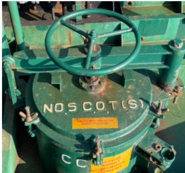
Figure 1: Enclosed space entry location with warning.
