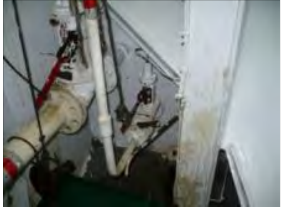
Quick closing valves INOP - tied open
