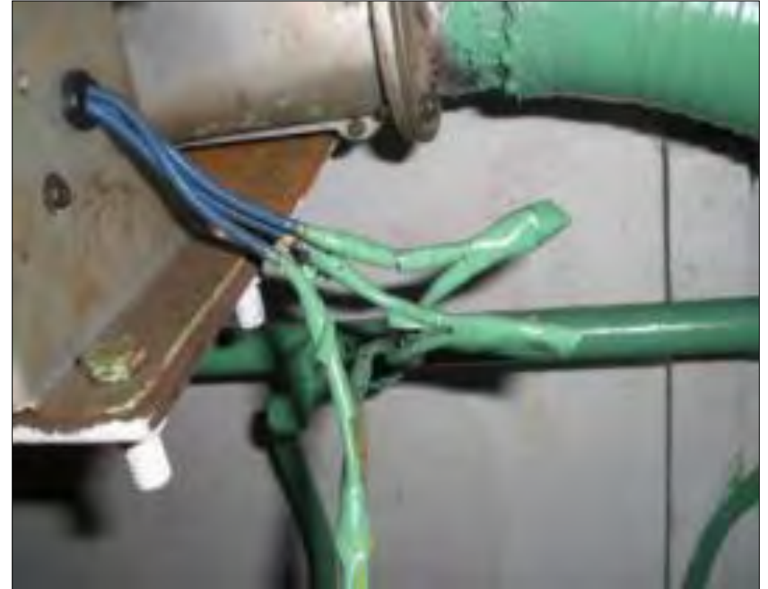
Loose electrical cables
